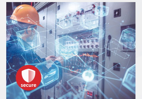
Reduce safety hazards in manual operations
